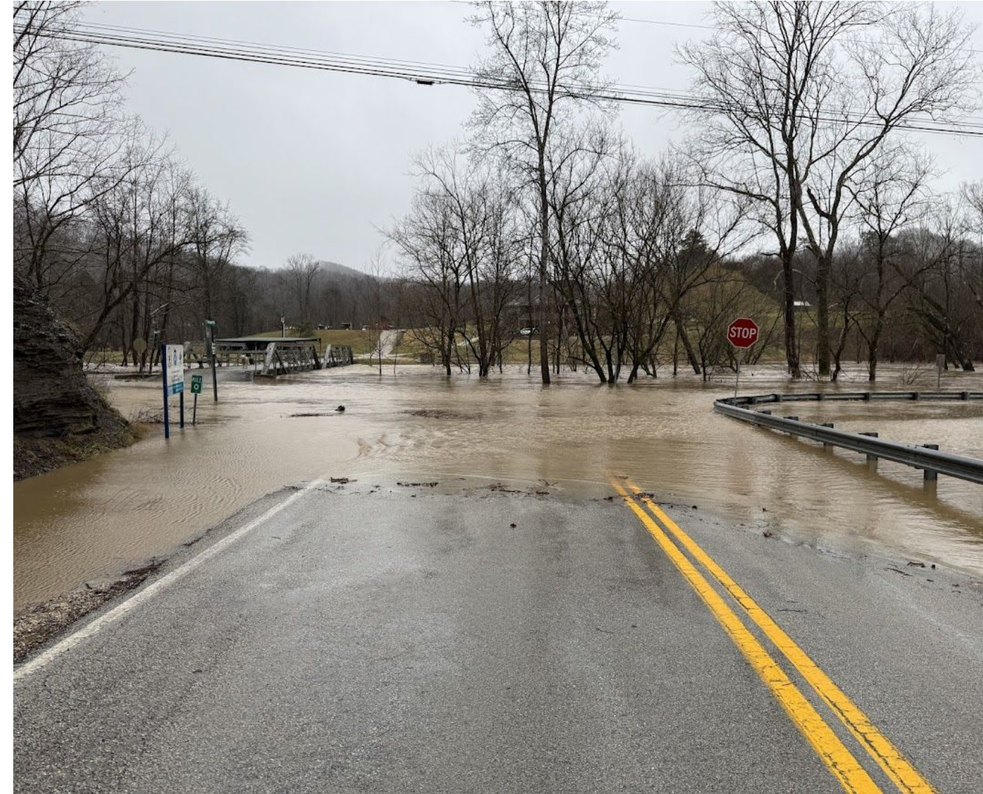
Flooding near the NWS office in Jackson, KY (February 16, 2025)
