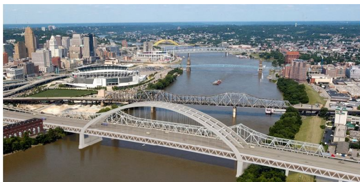
The rendering above depicts a new companion bridge across the Ohio River linking Cincinnati OH (at left) to Covington KY (at right), directly adjacent to the existing Brent Spence Bridge. The “tiered arch” design depicted is a preliminary concept.
